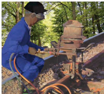
Figure 3.11 Thermit process for joining railway tracks
